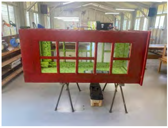
The second photo shows the telephone box freshly painted following replacement of rotted timberwork on the partly renovated project.
