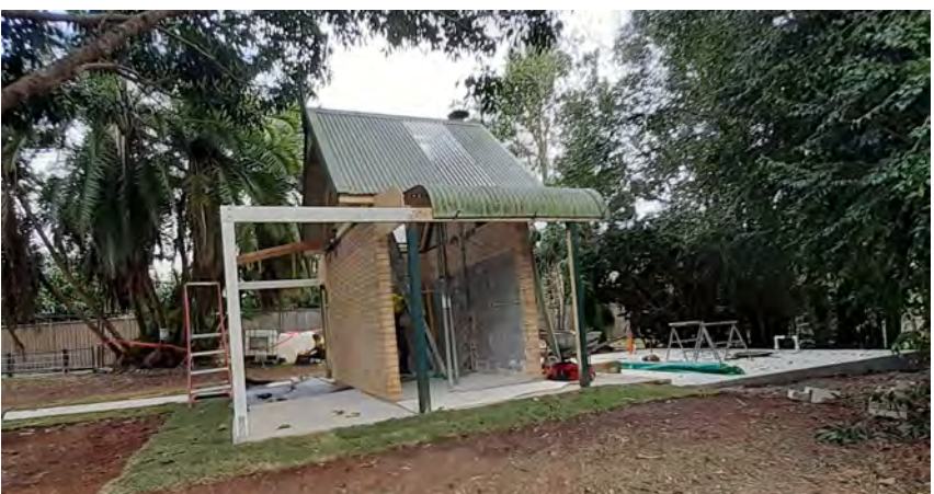
Old structure stripped, additional pad laid ... work in progress
